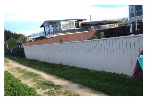
It was suggested that a small bund at the end of Tait St could be constructed to stop water flowing onto Tait St and Broadsea Ave from behind the wall. During Cyclone Fehi it was observed that this was the route that a lot of the flood water took onto Broadsea Ave.
