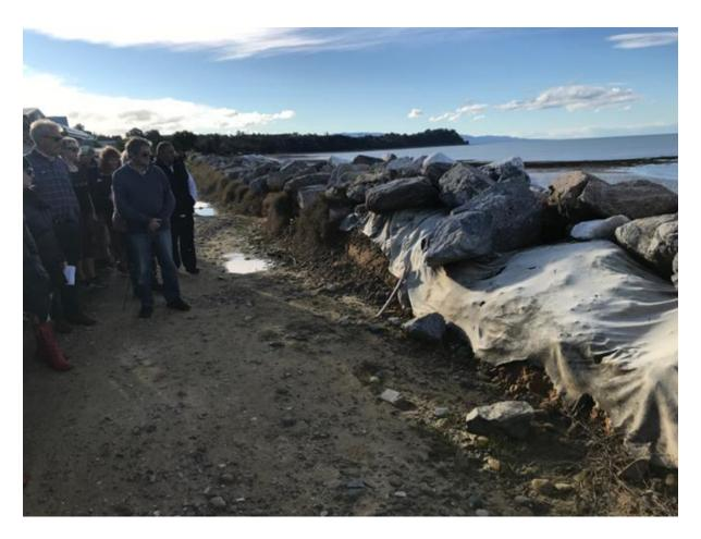
It was suggested that, if the part of the sea wall that extends above the walkway was made of large rocks with voids between, then water could flow through the seawall back down to the beach.
